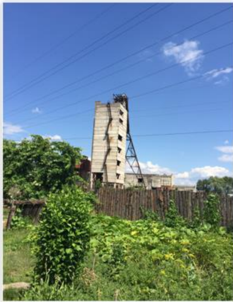
Figure: Skip Shaft of Mine No 9
