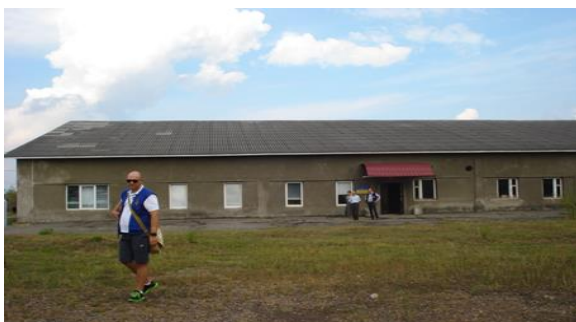
Figure 3.6.8: Central Mine Administrative building (part in use)
