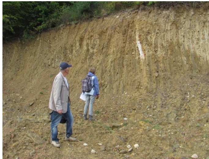
Figure 3.3.B.2: Weathered, deformed bedrock
