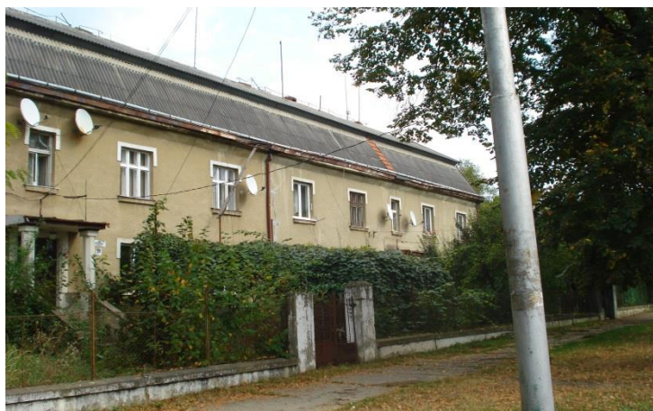
Figure 3.6.14: Outward aspect of the apartment building
