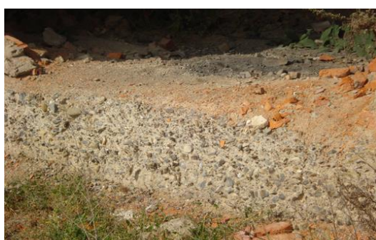
Figure 3.6.1: Unreinforced concrete platform
