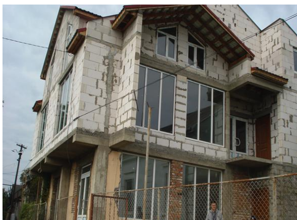
Figure 3.6.6: Building with mixed material masonry, some concrete elements and thin slabs
