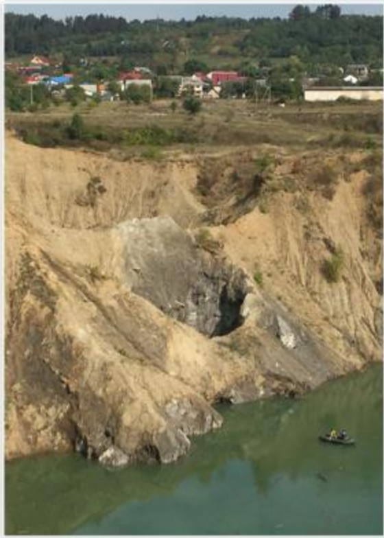
Figure: Crater of Mine No 7 during water sampling by the Ukrainian Mountain Rescue Team. The hole in front of the boat is the old mining shaft No 7.
