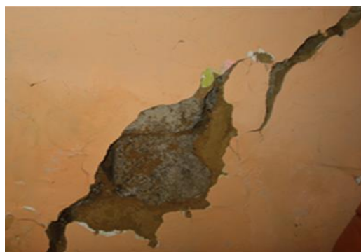
Figure 3.6.4: Plaster of compressed earth with straws
