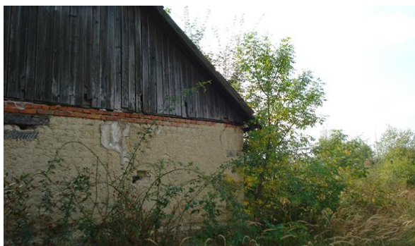
Figure 3.6.3: Masonry of wood, bricks and adobes without “chainage”
