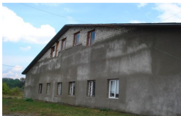
Figure 3.6.10: Central Mine Administrative building (east side)
