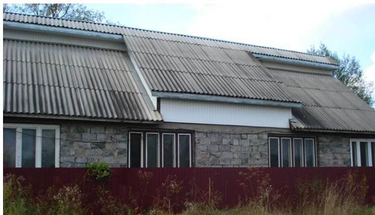
Figure 3.6.5: Roof covered by asbestos slates
