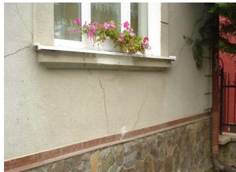
Figure 3.6.18: Masonry crackings
