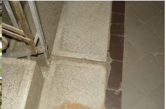
Figure 3.6.17: One of the three staircases
