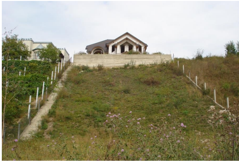
Figure 3.6.35: Retaining wall in the residential area near Tisza River
