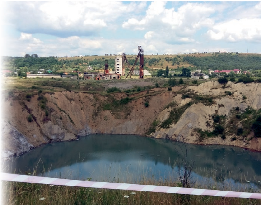
The abandoned Solotvino salt mine, with one of the craters in the foreground as a result of implosion and intrusion process of water.
