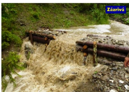
Figure 18 Ditch for overland flow, Slovakia ( http://nwrn.eu/measures-catalogue )
