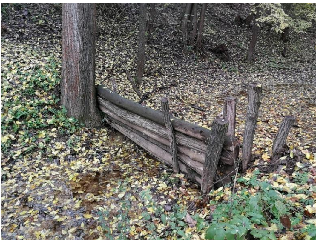
Figure 14 Log dam in Püspökszilágy ( https://life-climcoop.hu )
