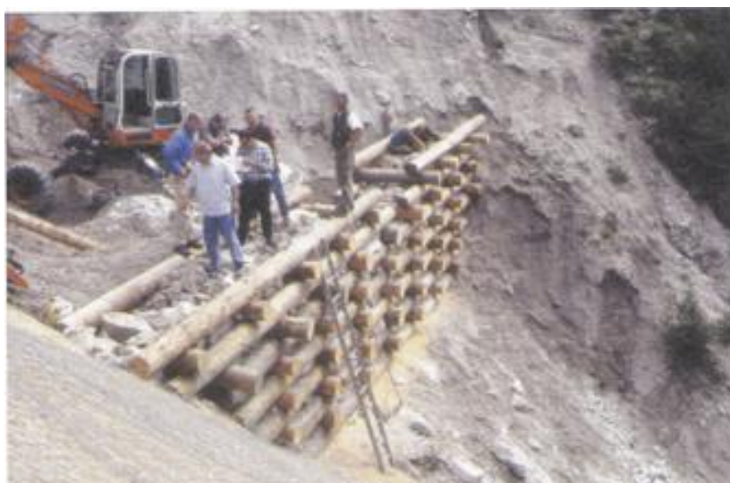
Figure 37 Construction of a wooden and stone dam (Malaguti 1993)
