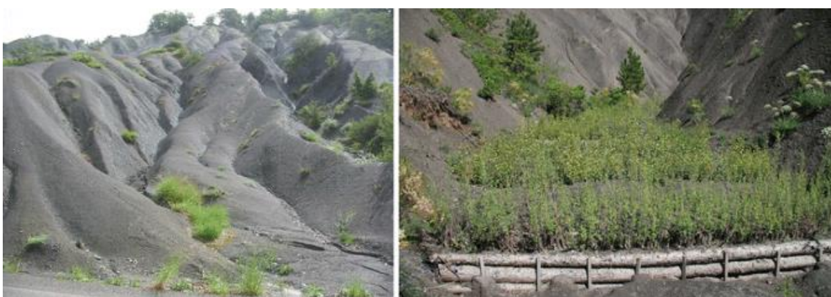
Figure 25 Brush layers and mats to stabilize marly gullies, French Southern Alps, France ( https://link.springer.com )
