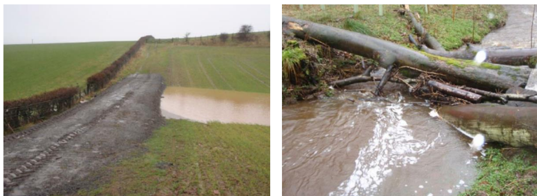
Figure 29 Woody debris and soil bunds, Belford, UK (Wilkinson 2010)
