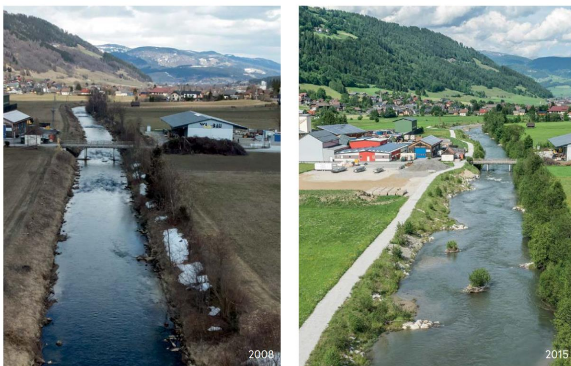
Figure 16 River widening and protective structures, before-after photos (FMST 2018)
