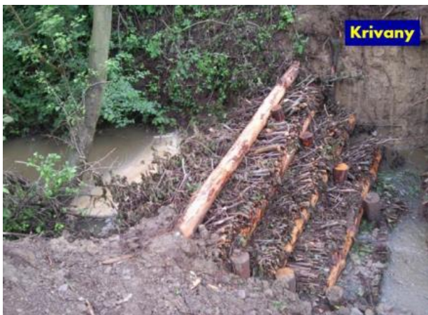
Figure 20 Sediment capture pond, Slovakia ( http://nwrn.eu/measures-catalogue )
