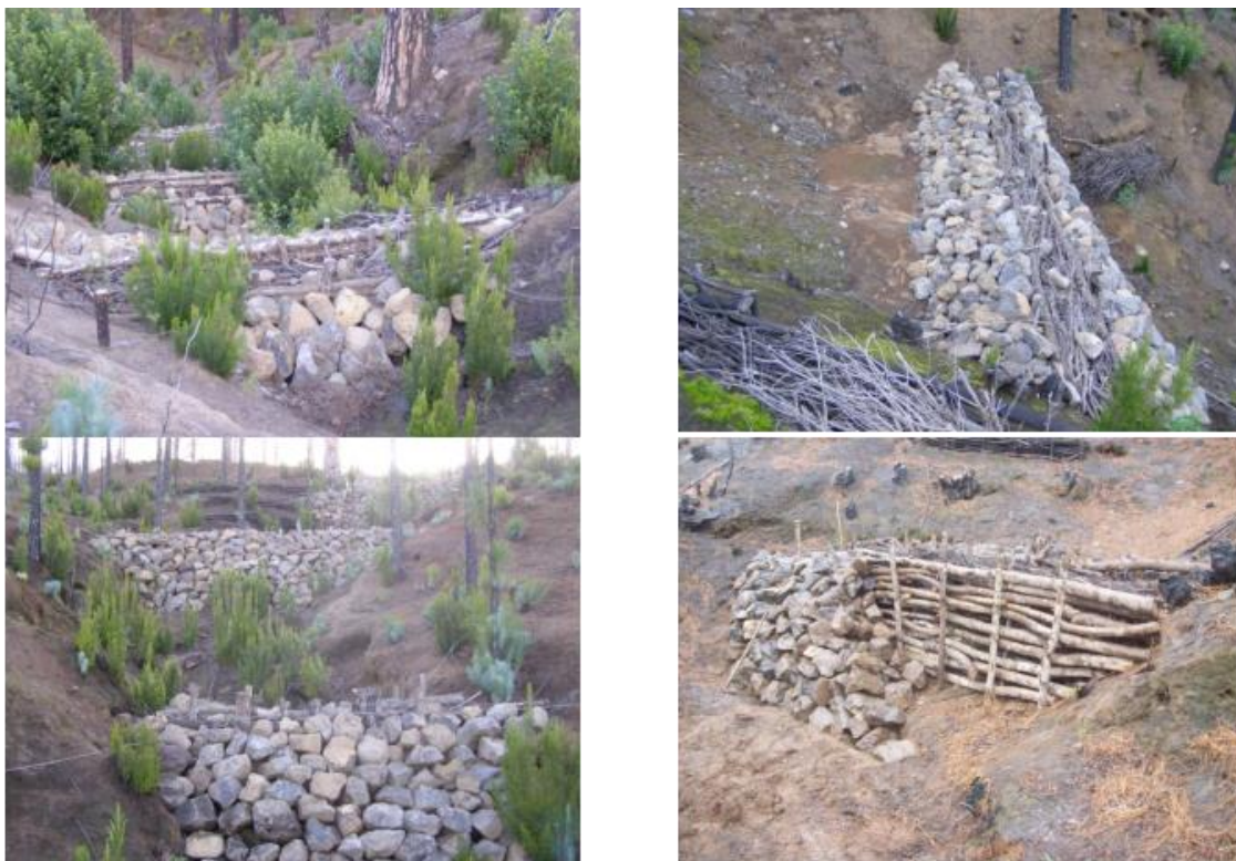
Figure 12 Gully control with dam (Tardío, García 2016)
