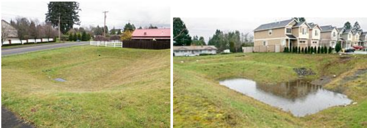
Figure 11 Grass infiltration pool ( https://www.stormwaterpartners.com )
