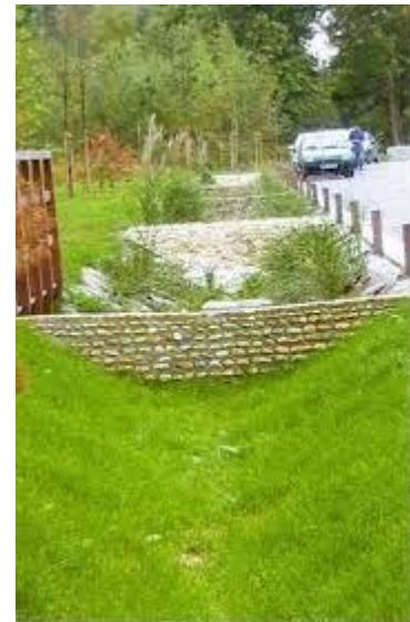
Figure 26 Stormwater retention basin ( https://crowd-geoikp.kajoservices.com )
