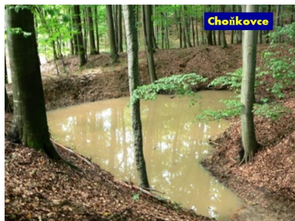
Figure 21 Peak flow control basin in forest, Slovakia ( http://nwrn.eu/measures-catalogue )
