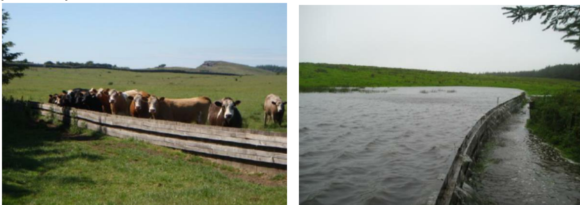
Figure 28 Wooden bund, Belford, UK (Wilkinson 2010)
