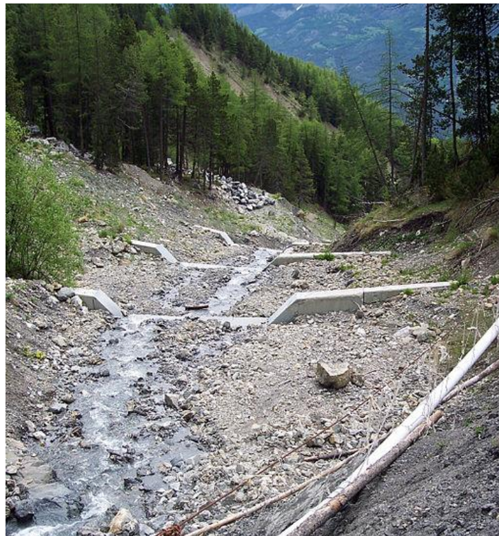
Figure 13 Gully bed stabilization / check dams ( https://www.appropedia.org/ )
