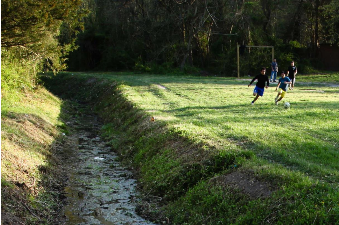
Figure 10 Grass drainage ditch ( https://www.chesapeakebay.net )
